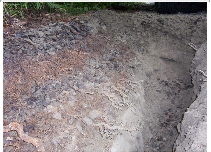
Massive amount of roots in cable covers for electrical wires, Stockholm Sweden.
