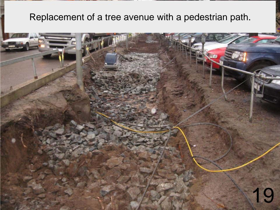
Soil only where the root ball will be placed. The rest of the ground filling is rocks in different fractions.
